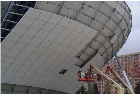
Figure 2: Double-curved cladding elements: Heydar Aliyev Cultural Centre (Baku, Azerbaijan)
