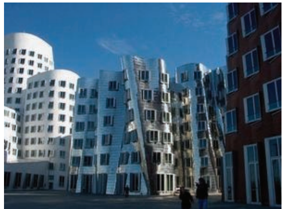
Figure 1: Double-curved load-bearing elements: Der Neue Zollhof' (Düsseldorf, Germany)
