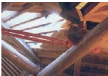
Fig.24 Steel anchor to fix round beams (Larsen O.P., 2008)
