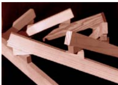
Fig.23 Wooden parts between beams, where they are fixed on (Larsen O.P., 2008)
