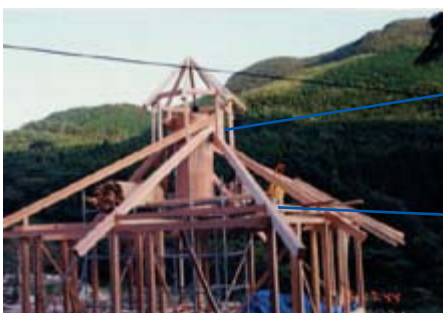
Fig.21 Joint using friction (Larsen O.P., 2008)
