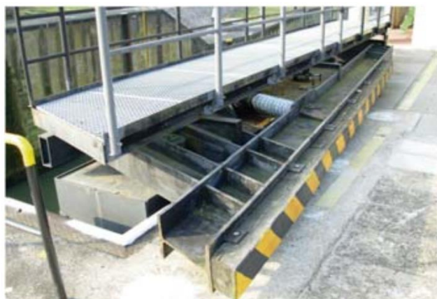
Figure 32: Ship collision absorber (InCom_Working_Group_151, 2014)
