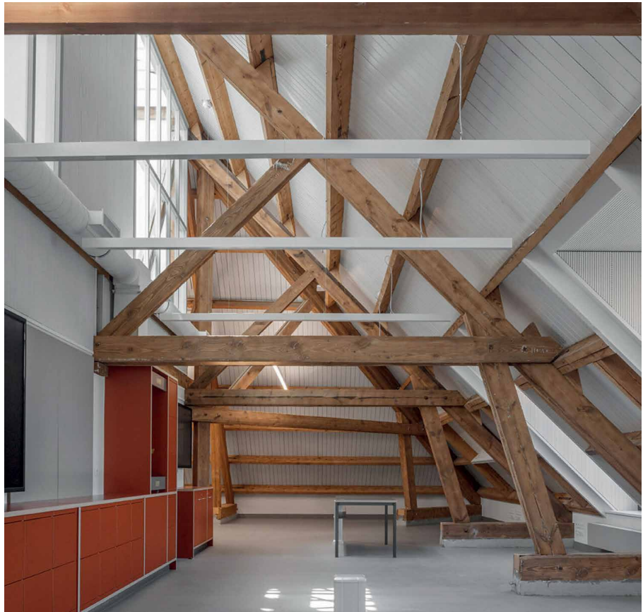
FIG. 4.10 Attic trusses at the old building of the Campus Cadix. Source: KSA
