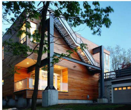
Big Dig House | Exterior
