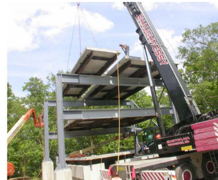
Construction of the building
