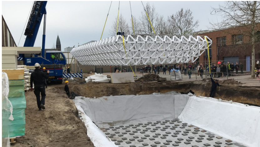
Figure 5.1: HoCoSto USTES being placed in a prepared insulated pit. The picture was taken at a project with a 250 m 3 USTES for a newly built school in Boekel. The USTES is part of a central heating and cooling system that is relying on solar collectors instead of the traditional natural gas.
