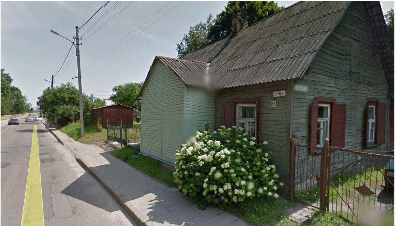
FIGURE 13. DUE TO INTENSE TRAFFIC, OLD HOUSE MAIN ENTRANCE, WHICH USED TO BE A REPRESENTATIVE PART OF BUILDING, COVERED WITH BLANK WALL. SOURCE: GOOGLE STREET VIEW
