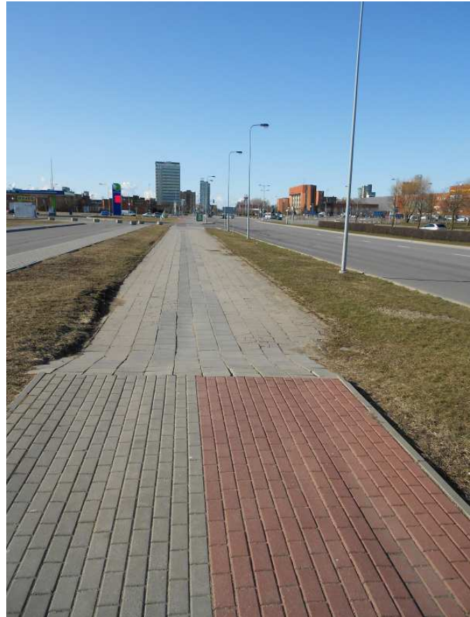
FIGURE 57. EXAMPLE OF DISINTEGRATED BICYCLE PATH DESIGN IN KLAIPĖDA, TAIKOS pr. BICYCLE PATH ENDS ALONGSIDE PROPERTY BOUNDARIES WHERE "RIMI HYPER MARKET" WAS OBLIGED TO PROVIDE BICYCLE AND PEDESTRIAN PATHS. BICYCLE PATH STARTS AGAIN ALONG PROPERTY BOUNDARIES OF "NESTE" GAS STATION, BUT ON THE OPPOSITE SIDE OF THE SIDEWALK. SOURCE: SUMODELIUOK LIETUVĄ
