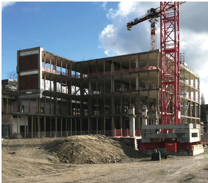
Figure 33. Structural re-use of the existing factory building. Image by BHSF Architekten.
