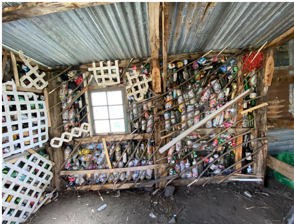
(c) Detail of the plastic bottles insulation
