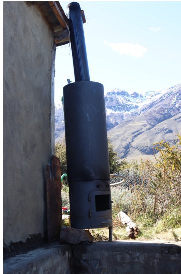
(c) Wood burning current water tank
