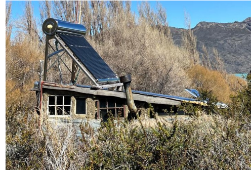
(b) Solar heated current water tanks
