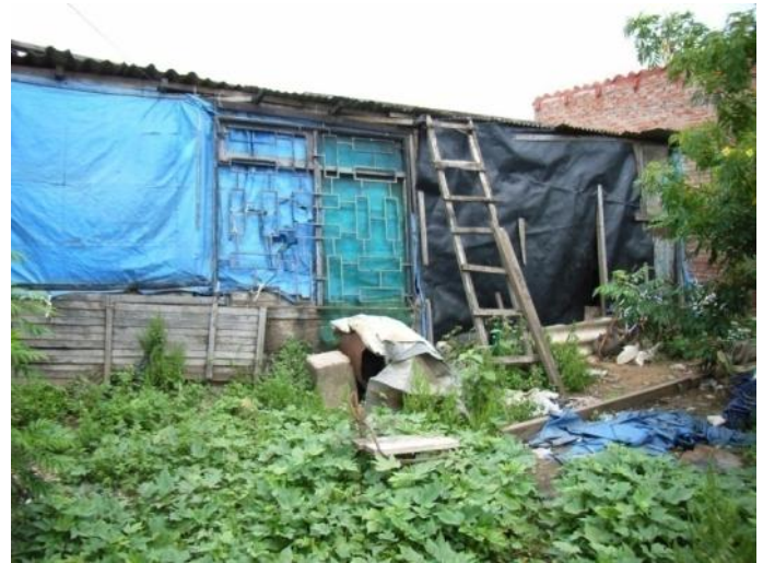
Fig. 2.10 Construction made out of loam, sheets of corrugated iron and plastic cloths.
