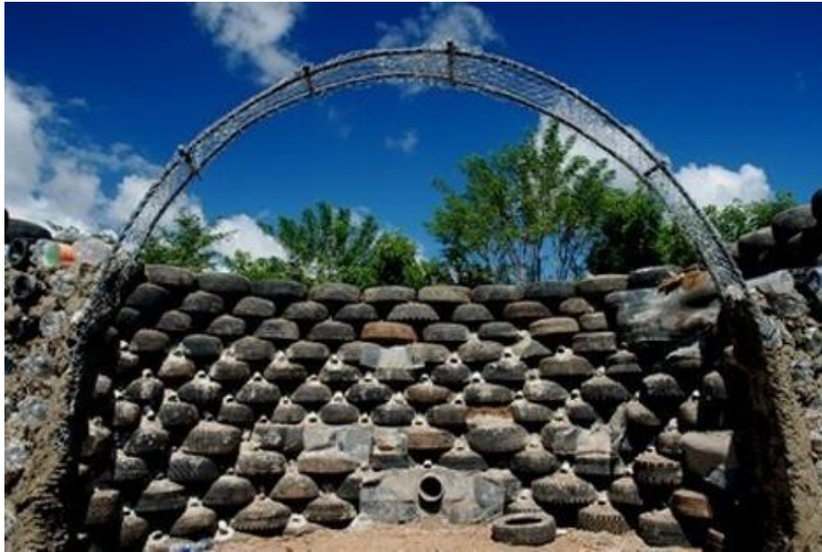
Fig. 3.3 Earthship, construction with car tires
