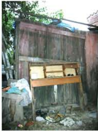
On the left the old kitchen which is located behind the first construction. This kitchen is no longer in use, because of the large number of holes in the roof.
