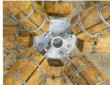
Fig. 4.11 Consolidation of the round wood joint
