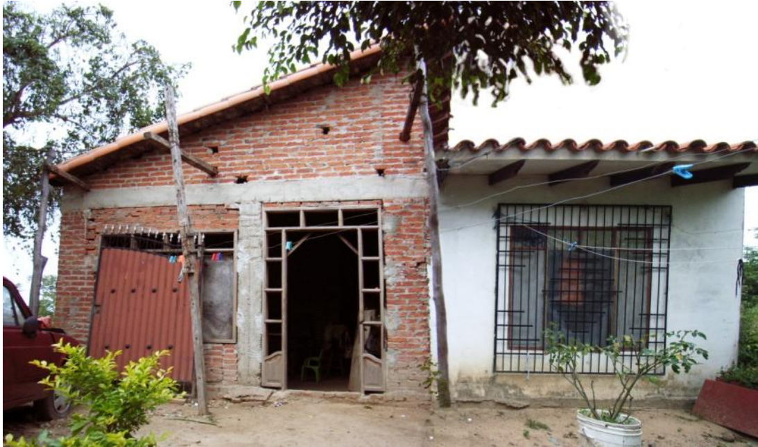
Fig. 2.8 Self constructed brick house in Santa Cruz de la Sierra.
