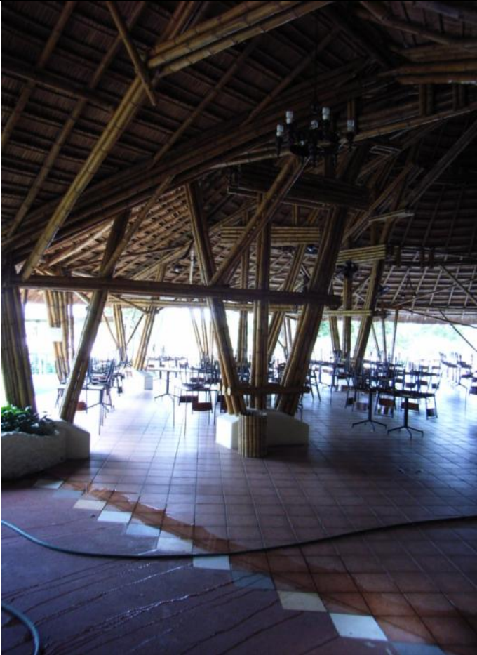
Fig. 2.14 Bamboo constructed restaurant "Casa del Camba" in Santa Cruz de la Sierra
