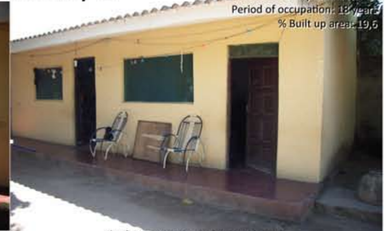
The first two constructions made with bricks and steel plates. They are used as bed rooms.
