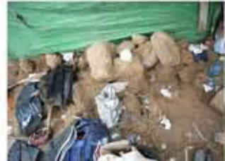
A fallen adobe wall
