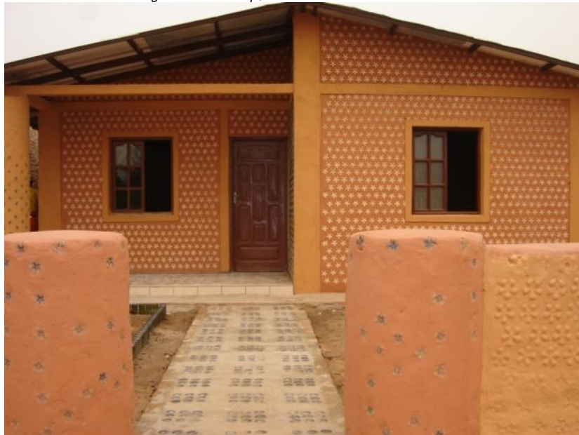
Fig. 3.4 "Casa de botellas", construction with plastic bottles
