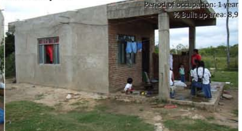
The owner rents his house to this family until the house is finished
