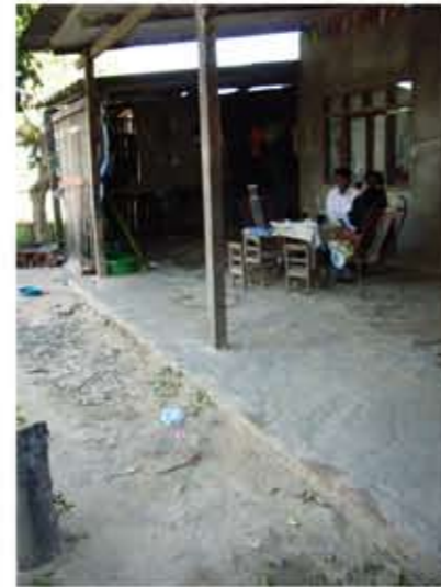
The "galleria" with a cement floor.
