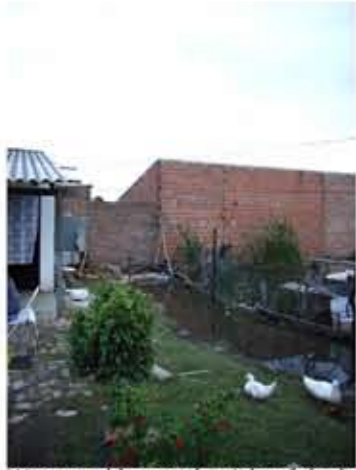
Water problem to the right of the house
