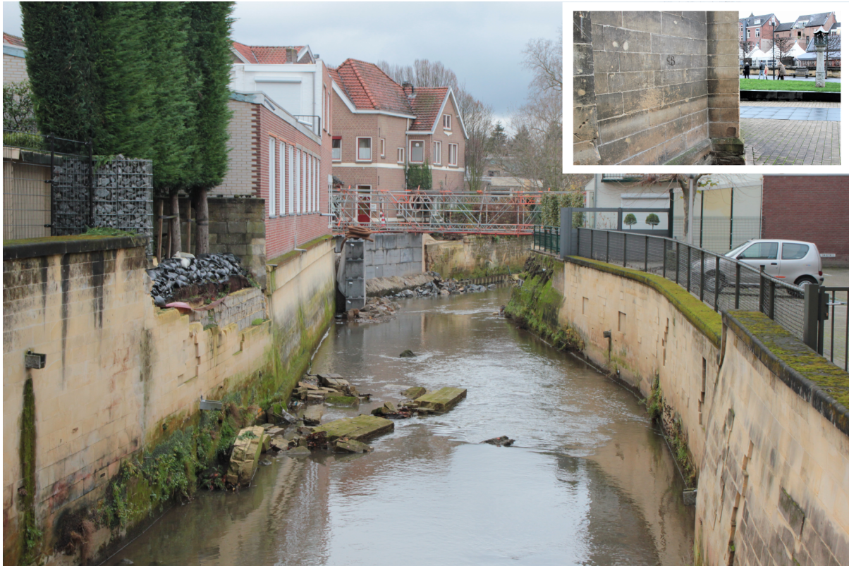
Figure 2.7: The main channel of the Geul in the centre of Valkenburg, limited in its course by retainment walls and buildings. In the background, a temporary bridge has been constructed since the original bridge of the Emmalaan was destroyed. Although the picture was taken on 11-02-2022, 7 months after the event, the water level of the flood event is still vaguely visible on the marl walls, as can be seen on the top right corner picture. Both pictures have been taken by the author of this research.
