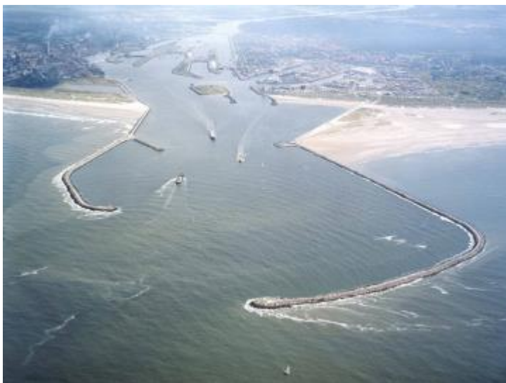
Figure 1.1: The IJmuiden breakwaters as seen from above [Ref. 4]
