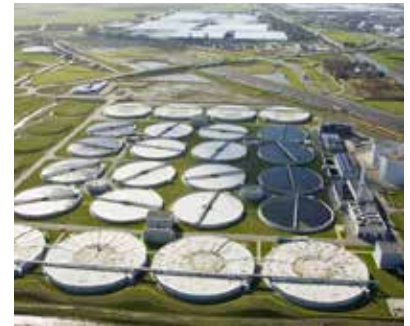
Figure 7.6. Water Treatment plant Harnaschpolder (Zoethout, 2015).
