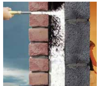
Figure 10.17. Insulation method of the cavity-wall. Source:
