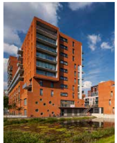
Figure 7.8. New buildings in the Poptahof (RVO, n.d.).
