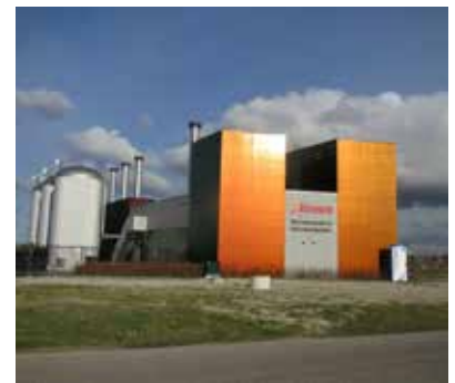
Figure 7.7. Heat station Harnaschpolder (Harnasch foto, 2012).
