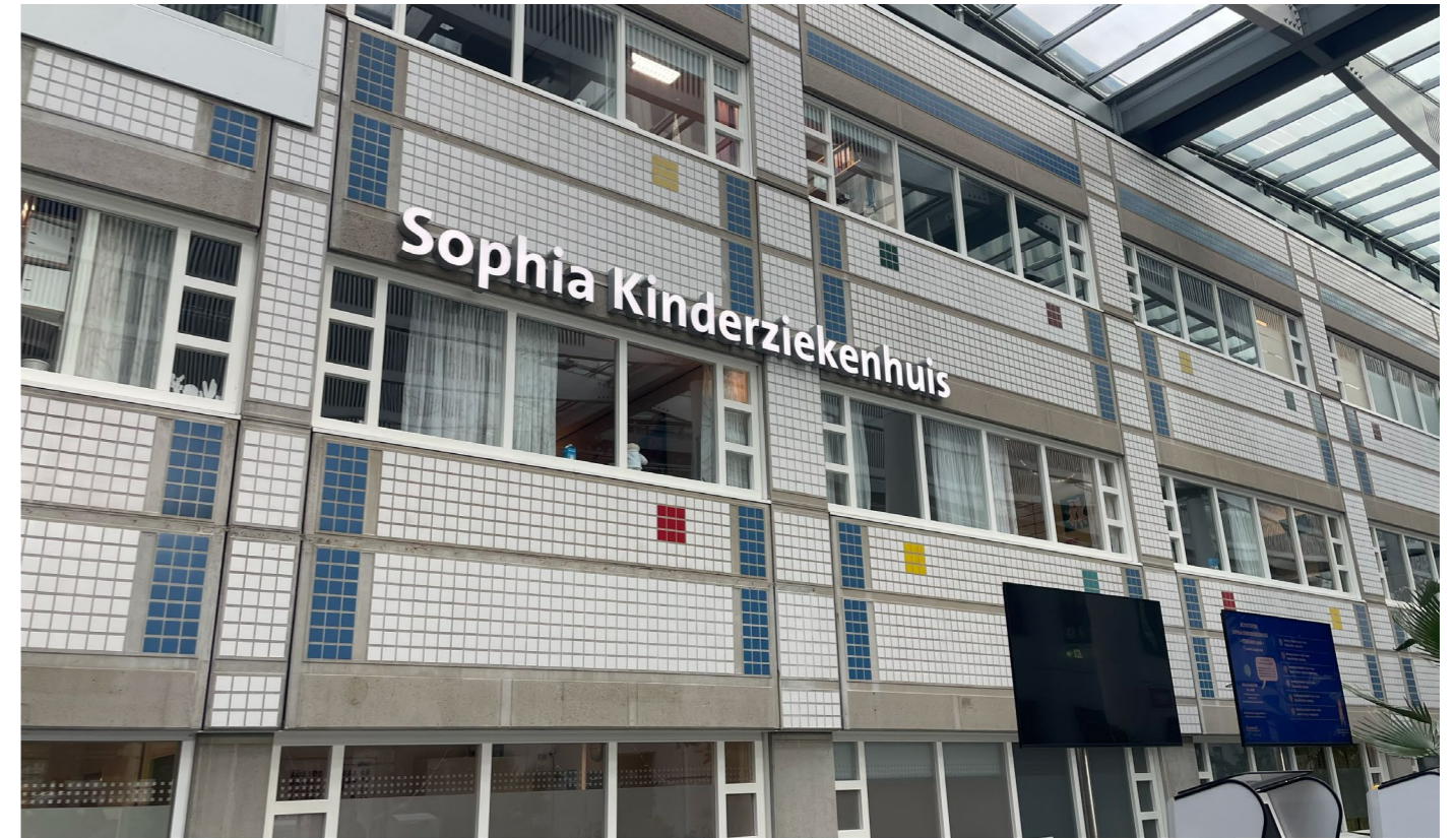
Figure 4: Entrance Hall Sophia Kinderziekenhuis
