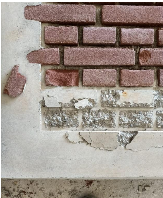
Figure 6.12: Brick damage and concrete damage
