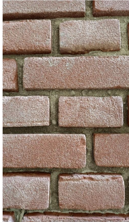
Figure 6.11: Joints between the bricks where silver-sand has been applied in the correct way
