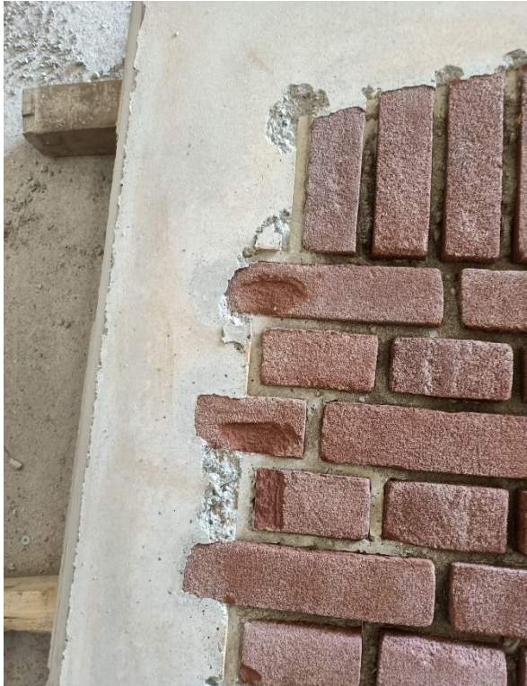
Figure 6.10: Damages in the concrete on the edges of the bricks
