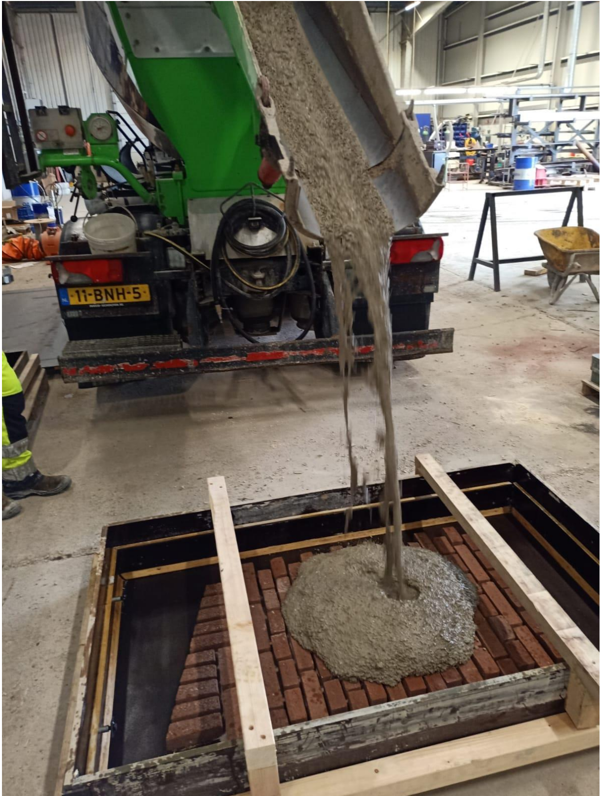
Figure 5.2: Pouring the concrete with the mixer truck
