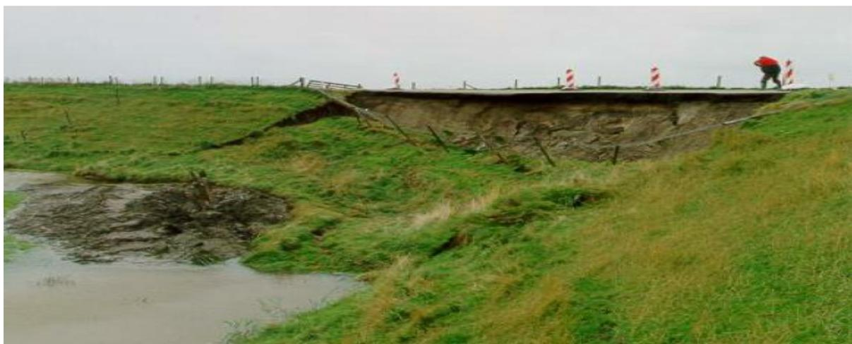
*Figure 3: Slip circle due to loss of macro stability (GeoDelft, 2007)*
