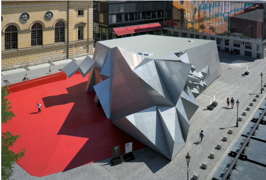
Fig. 7.3: "Our strategy to achieve soundscaping comprises three steps: Firstly, to realize the shielding effect between square and street, secondly, to shape the geometry of the Pavilion in such a way that the surface deflects noise, and thirdly, to design the surface of the Pavilion in such a way that it reflects and absorbs sound. In order to implement the objectives of the interior spatial acoustics, the interior wall and ceiling surfaces were fitted with a combination of perforated absorbing and smooth reflecting sandwich panels." (Coop Himmel(l)au, 2010)
