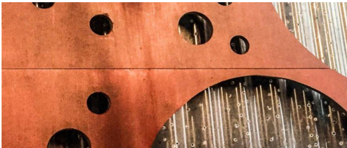
Fig. 7.4: The intention of this proposal was to "strengthen the effect of multiple reflections and absorption by a double layer façade structure. The irregular distribution of the holes intended a division in transparent or less transparent parts of the façade. For the second layer between the outer layer and the wall, a transparent wave formed polystyrene roof cladding was used. Distributing through the wave formed surface will reduce the direct reflected sound energy. In addition to this, extra holes in the surface were drilled in order to improve the absorption properties of the façade element". Source: Acoustically effective façades design (Krimm, J., 2018: 173)
