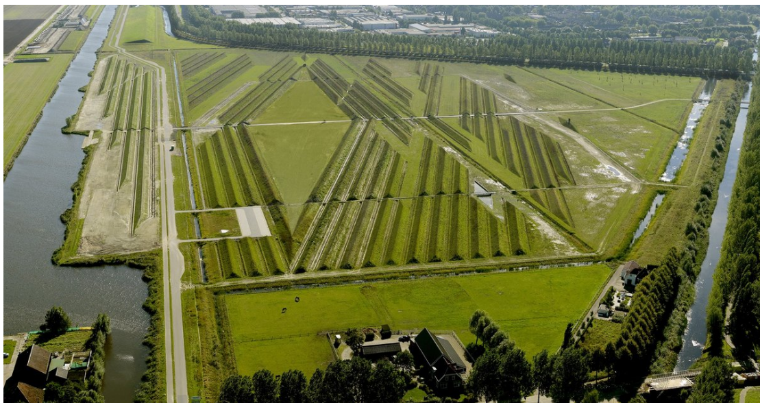
Fig. 7.2: On the authority of Schiphol a multidisciplinary team worked on a world first project: a park that exists by the grace of low frequency ground noise caused by aircraft taking off. Because of its design, the park landscape contributes to a considerable noise reduction. Measurements and calculations have shown that the ground noise is distorted and dispersed, as it were, by oblique planes.
