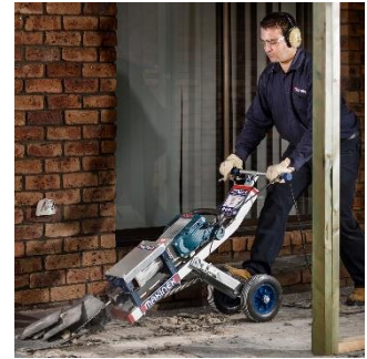
Figure 2: The jackhammer trolley in use.
