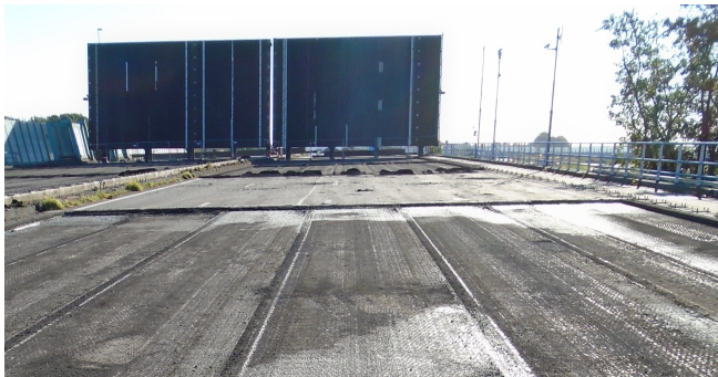
(a) Asphalt removed by asphalt ripper (span 4 is shown in the foreground, southern side is on the right)
