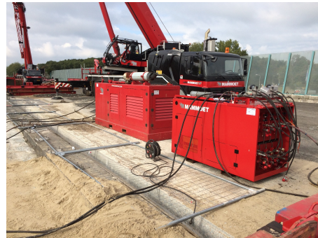
(b) Hydraulics for jack and power generator
