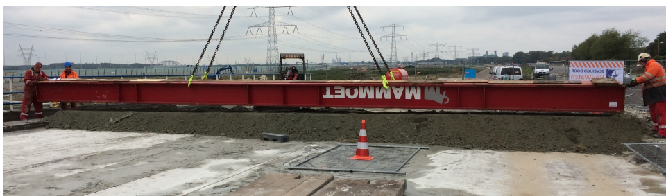
Figure 6.9: Steel bridge support beam placed on sand filling
