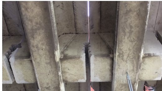
(b) Sawing and cylinder drilling through the cross-beams
