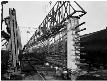
(a) Prefabrication of T-beam on-site
