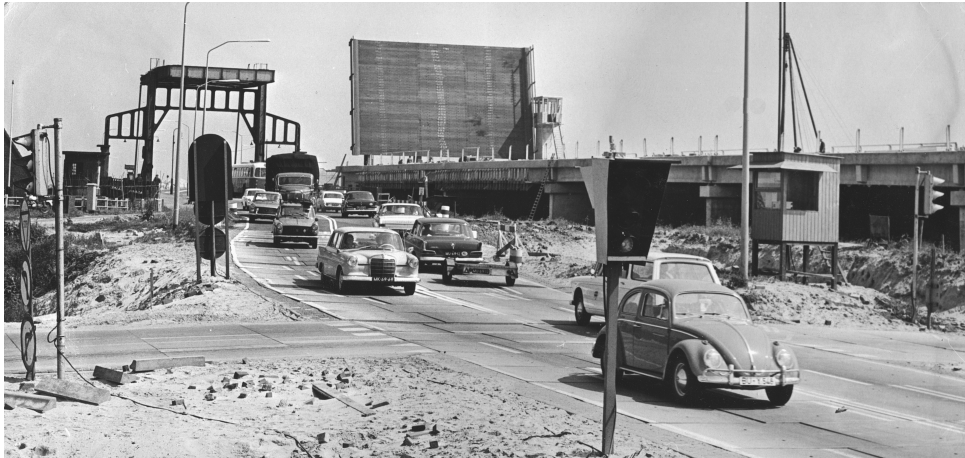
Figure 5.1: Construction of the new Vecht bridge in 1962 (right), existing bridge (left) (Rijkswaterstaat 2020)
