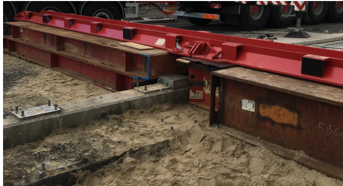
Figure 6.10: Steel bridge support beam(s) placed on sand filling and gap between the northern and the southern bridge filled with smaller steel work
