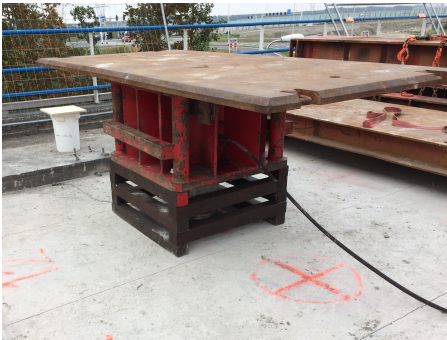
(a) Hydraulic jack (6000 kN) and steel plate supported by jacking timbers
