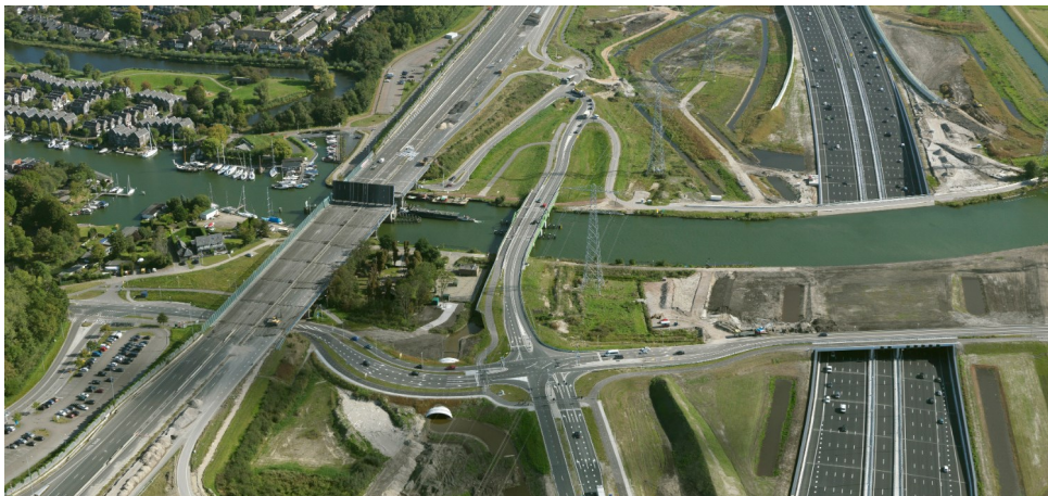
Figure 5.2: Completed new aqueduct (right), decommissioned Vecht bridge with opened bascule bridge prior to its demolition (left) (Rijkswaterstaat 2020)
