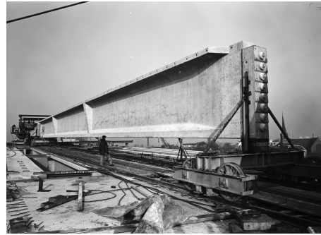
(b) On-site transportation of prefabricated T-beam using railway track
