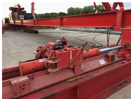
(b) Detail of jack inside sliding track
