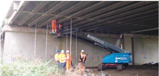
Figure 6.23: Use of mobile manlift (attaching equipment for test 1)
