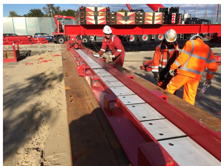
(a) Sliding track lined with teflon blocks
