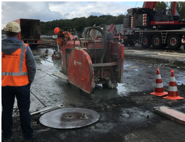
(a) Sawing through the integrated deck slab
