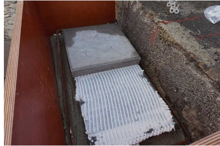
(b) Partially filling with concrete tiles
