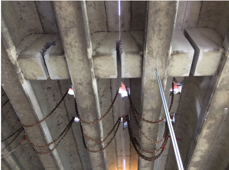
(b) Chains around T-beams (bottom side)
