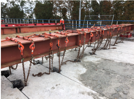
(a) Static steel beam with chains (top side)
