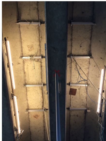
(b) Relative vertical slab deformation (loaded beam in the middle)
