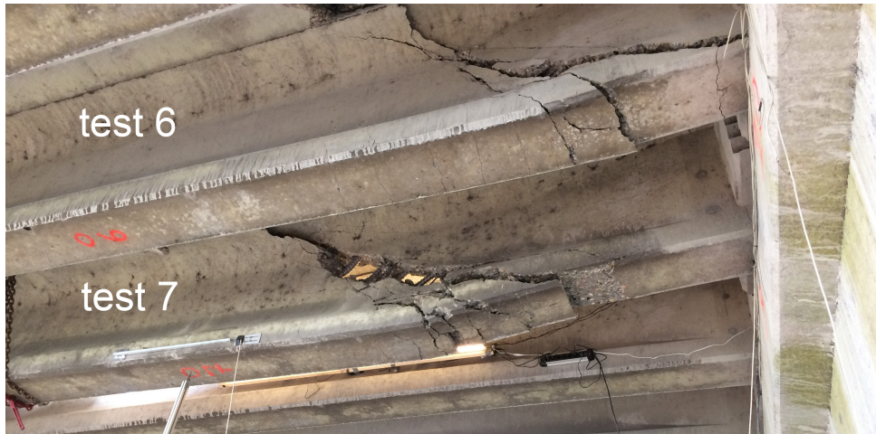
Figure 6.46: Flexural shear failure T-beam test 6 (top) and test 7 (bottom)
