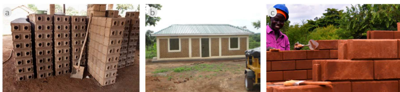
Figure 4. Earth bricks used in Uganda: (a) storage of CSEB in Jinja (‘Tanzania’ Brick); (b) house built with ISSB of Hydraform; (c) house under construction with Hydraform ISSB. Source: (a) Bredenoord, (b) Hydraform Uganda, (c) HYT Uganda.
