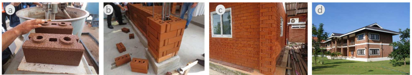
Figure 8. Housing solution with ISSB in Thailand: (a) ISSB of TISTR Thailand; (b,c) wall building with ISSB; (d) model house built with ISSB. Sources: (a–c) Bredenoord, (d) TISTR Thailand.
