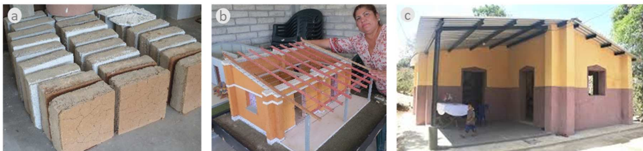
Figure 12. Adobe housing in El Salvador; (a) storage adobe blocks, (b) model earthquake resistant house, (c) built earthquake resistant house. Sources: (a) and (b) Bredenoord; (c) Fundasal.
