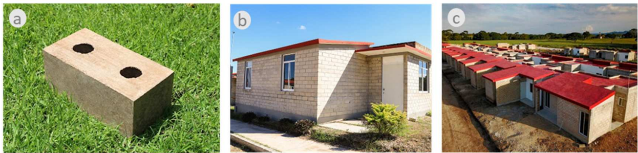
Figure 11. CSEB and housing in Mexico; (a) used CSEB, (b) built house, (c) realised Echale neighbourhood. Source: Echale.
