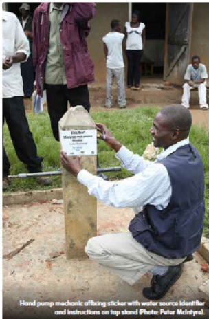
Figure 25. Handpump mechanic affixing sticker with unique water point identifier and instructions.
