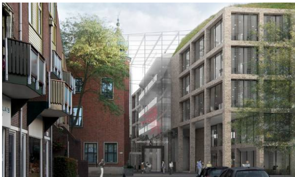
City hall by Kraaijvanger-Urbis (2011).
