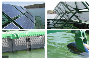
(b) Interconnected pontoons [11]
