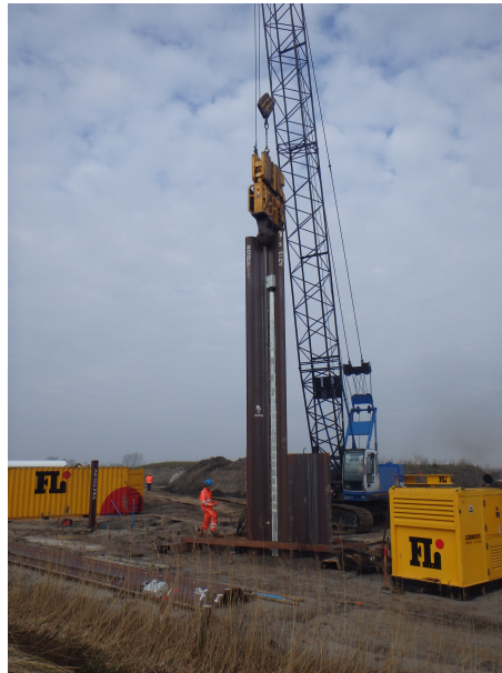
Figure 4.6: Installing of a sheet pile equipped with monitoring devices.
