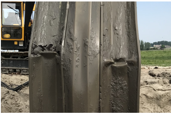
Figure 7.51: Excavated GU8N FST
