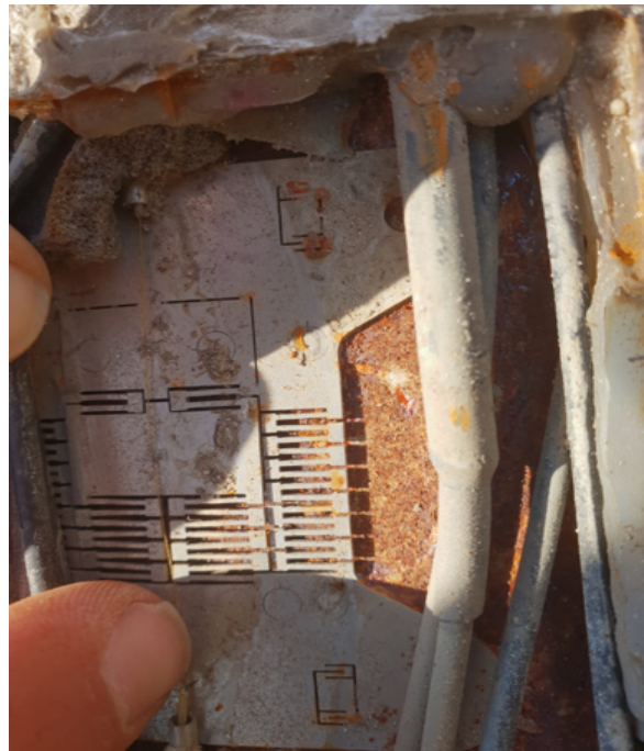
Figure 5.29: FBG sensor after test
