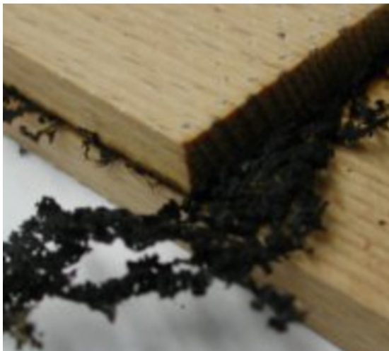
Figure 3.4 Welded wood connection with pushed out wood fibres. Laboratory for Timber Construction, IBOIS. (n.d.).
