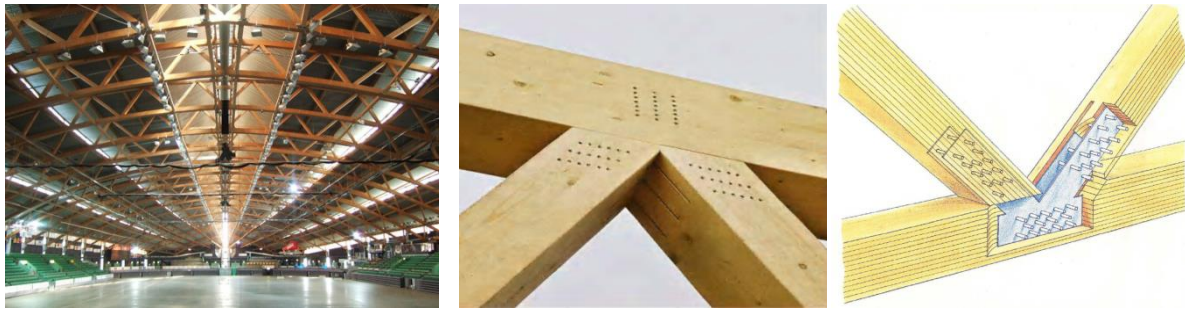
Figure 1 – Truss node with slotted-in steel plates (Kobel, 2011)
