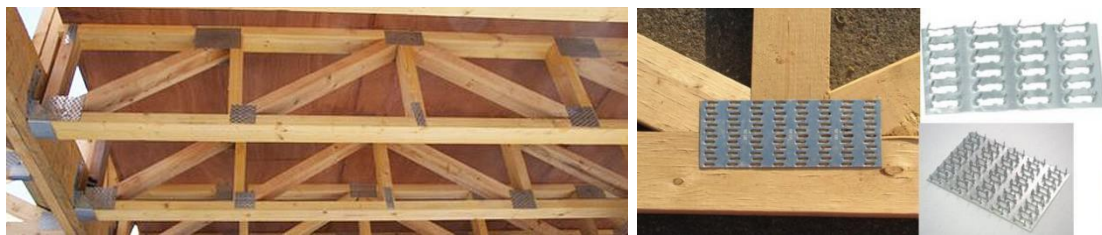
Figure 2 - Roof truss with punched metal plate fasteners (Hansson, 2001)
