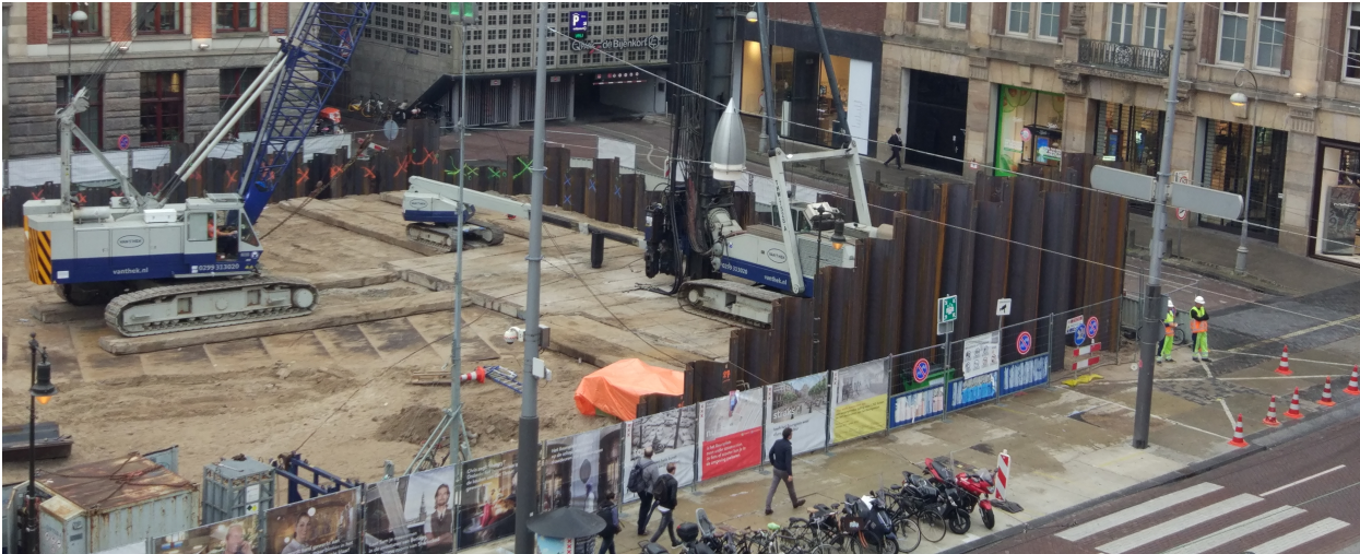
Figure 2: Bicycle parking garage Beursplein Amsterdam (CRUX, 2017)
