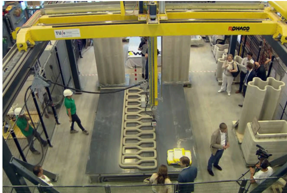
Figure 12: 3D printed concrete bicycle bridge (NOS, 2017)
