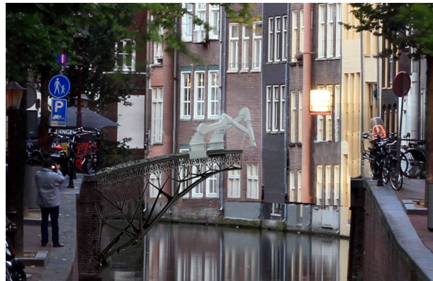
Figure 13: 3D printed stainless steel bridge (3dprimeur, 2015)
