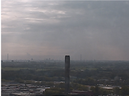
Fig. 9. Measured static target: Industrial chimney situated 1185 meters away from the sensor.
