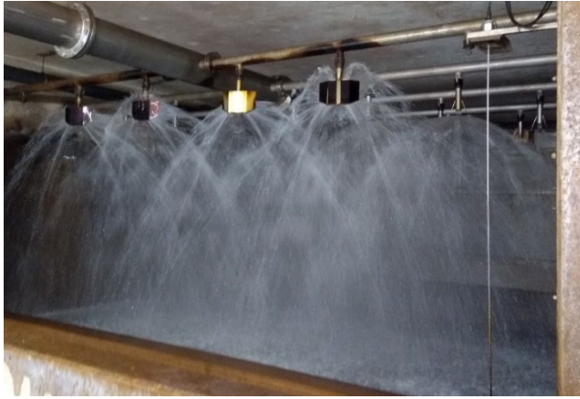
Figure 8. Spray aeration on top of the sand filter is one of the standard methods to introduce oxygen into anaerobic groundwater. Picture taken from drinking water treatment plant Leidsche Rijn (Vitens N.V.).
