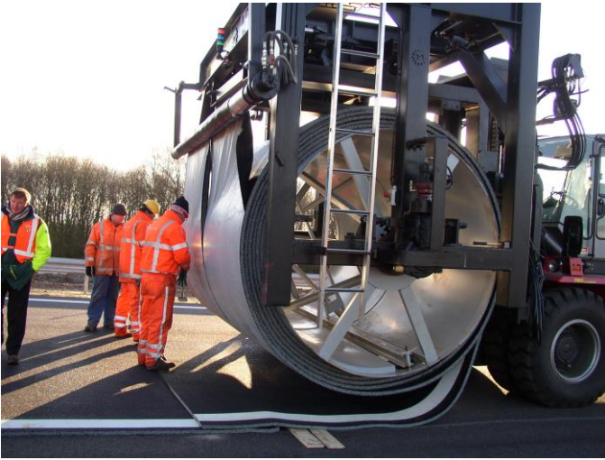
Fig. 4: Rolled up asphalt concrete
