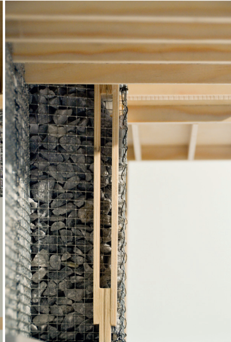
gabion boxes and harvested wood
