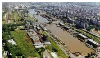
Puerto Madero before works
