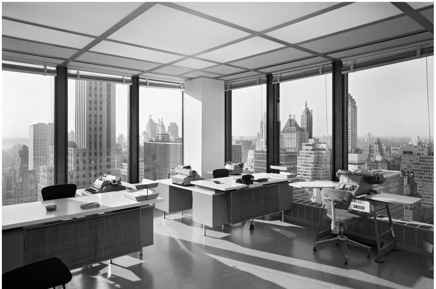
Figure 05 Uninsulated single-paned curtain wall on a typical office floor at the Seagram Building In New York.
