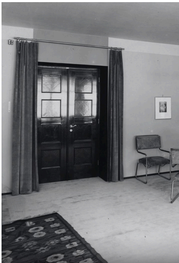
Figure 08 Portiera reduces heat loss and prevents cold air entering the room when the doors is opened (1931).
