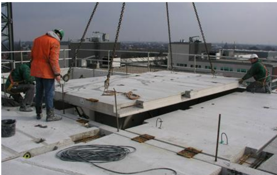
Figure 21 Massive concrete floor slabs [Hurks group, 2012]
