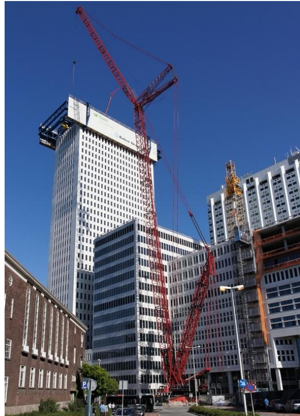
Figure 25 Dismantling of the Erasmus hoisting shed [Topaas, 2011]
