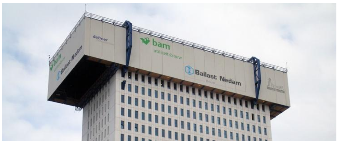
Figure 27 Hoisting shed at the Erasmus MC tower
