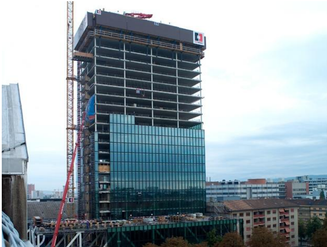
Figure 37 Automatic climbing formwork platform from Doka Group [Doka, 2012]
