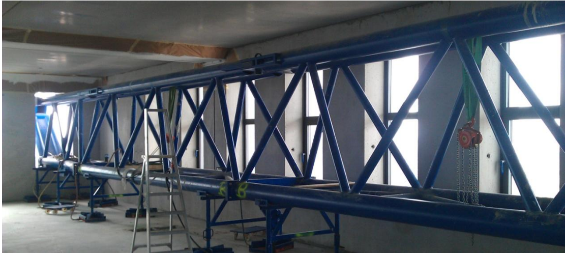
Figure 26 Supporting truss of the Erasmus MC tower
