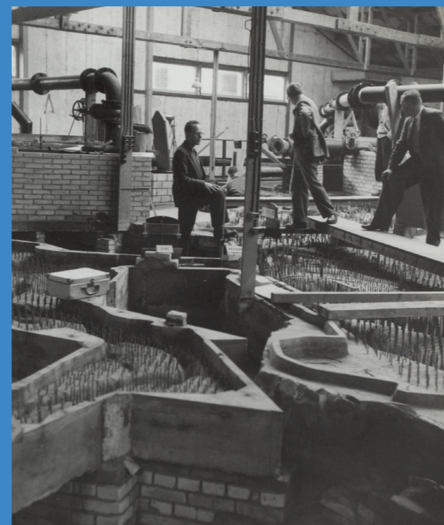
Figure 4.5: Scale models of the Deltawerken, Waterloopkundig Laboratorium Delft
