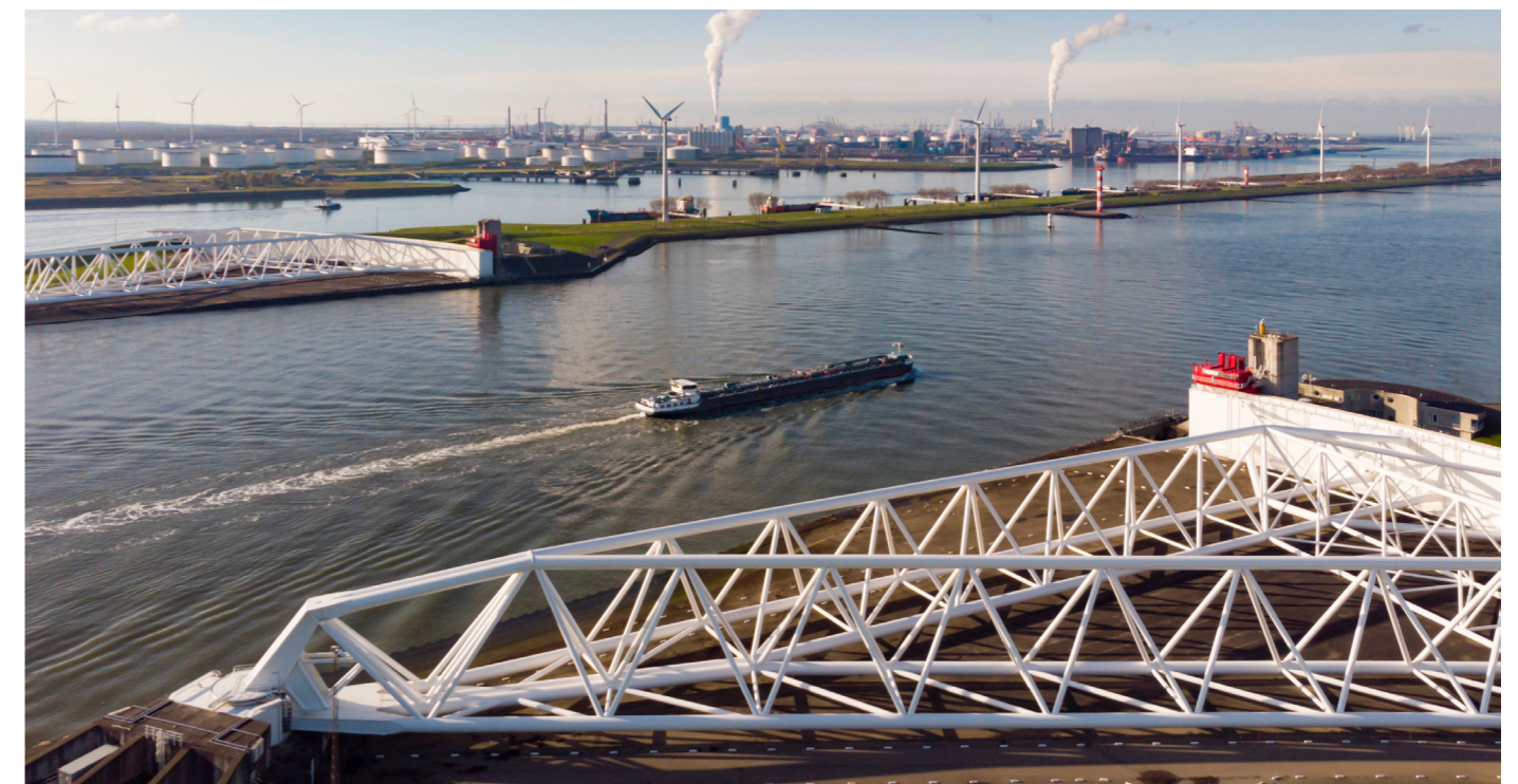
Figure 4.10: The Maeslantkering, the construction of which marking the institutional endpoint of the collaborative design capacity the Deltaschool had cultivated
