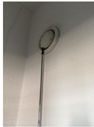
Figure 37: Fixed air velocity meter
