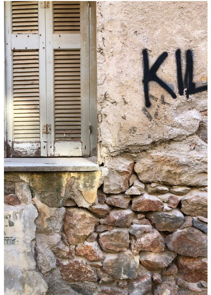
NORTH FACADE: LIMESTONE WALL WITH PLASTER COAT
