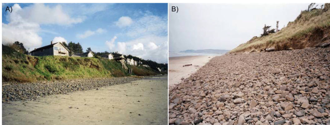
Figure 2.3: Dynamic revetment at Cape Lookout State Park, Oregon
