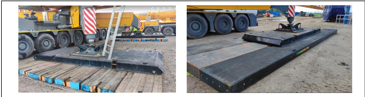
Figure 1: Load spreading mitigation measures
