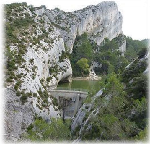
Figure 1: Glanum Dam was built in 1st century BC by the Roman Empire. Located in the southern France, the first ever built arch dam stored water for the Glanum Town. A new modern structure was built on top of the ruins and forms the Peiròu Lake (“Glanum Dam - Alchetron, The Free Social Encyclopedia,” n.d.)
