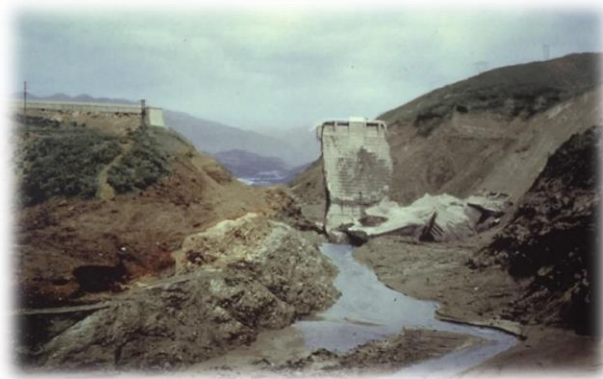
Figure 7: Picture of the Dam site after failure looking downstream (Rogers, 2013)
