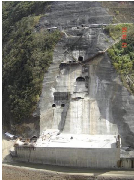
Figure 25: Shear key completed for Pirris Dam (Kanji,2017)
