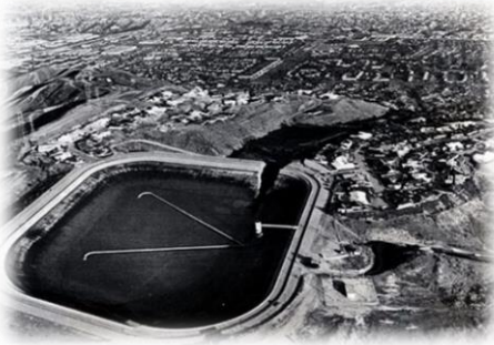
Figure 17: Aerial view on the Baldwin Hills Reservoir when it collapsed (MacDougall, n.d.)
