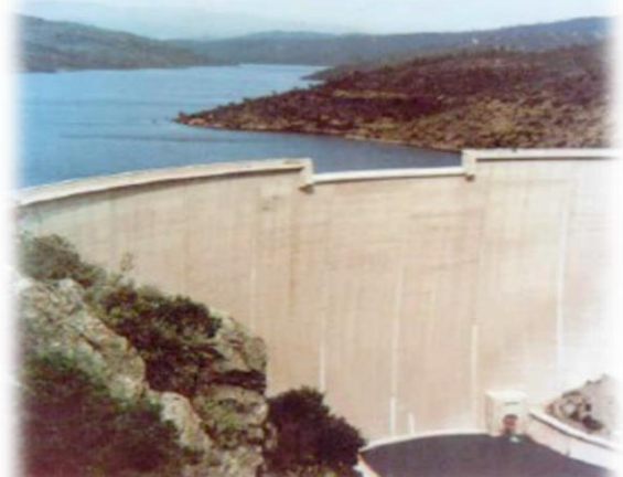
Figure 11: Malpasset Dam in 1954 (Goodman, 2013)
