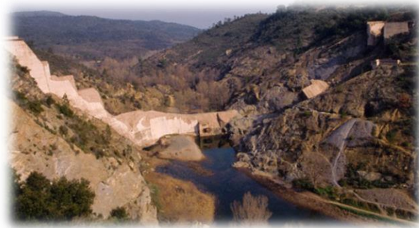
Figure 15: Malpasset Dam site after the failure (Goodman, 2013)
