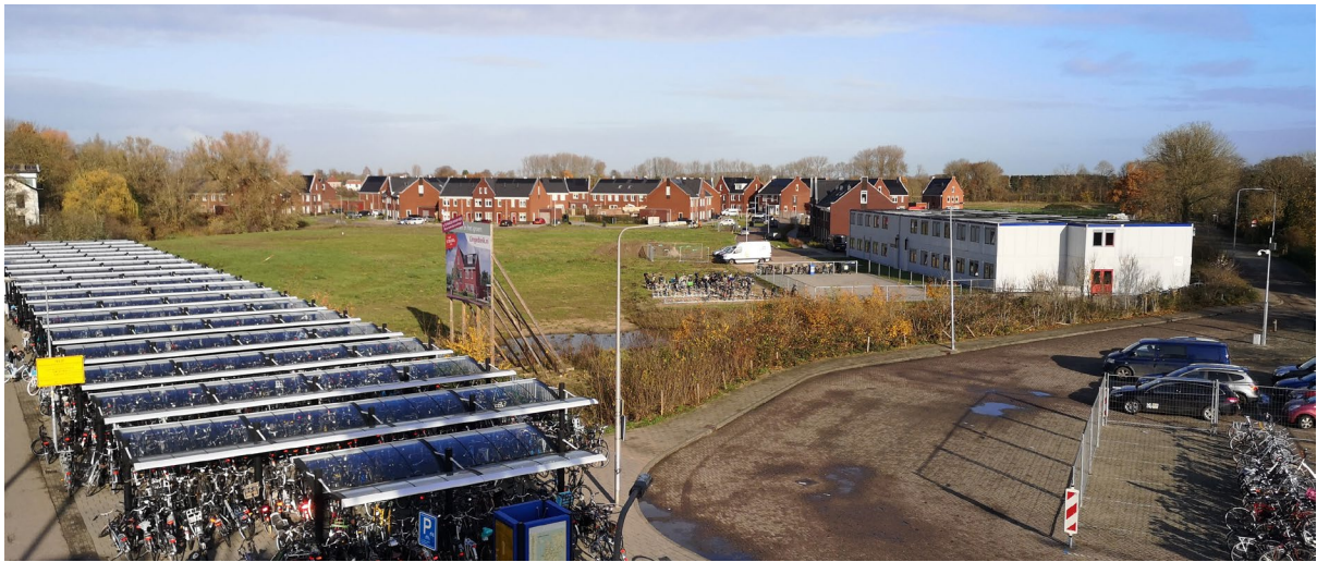
1 fig. 6.3.1: project location seen from bridge towards trainstation, with newly built family homes in the background
