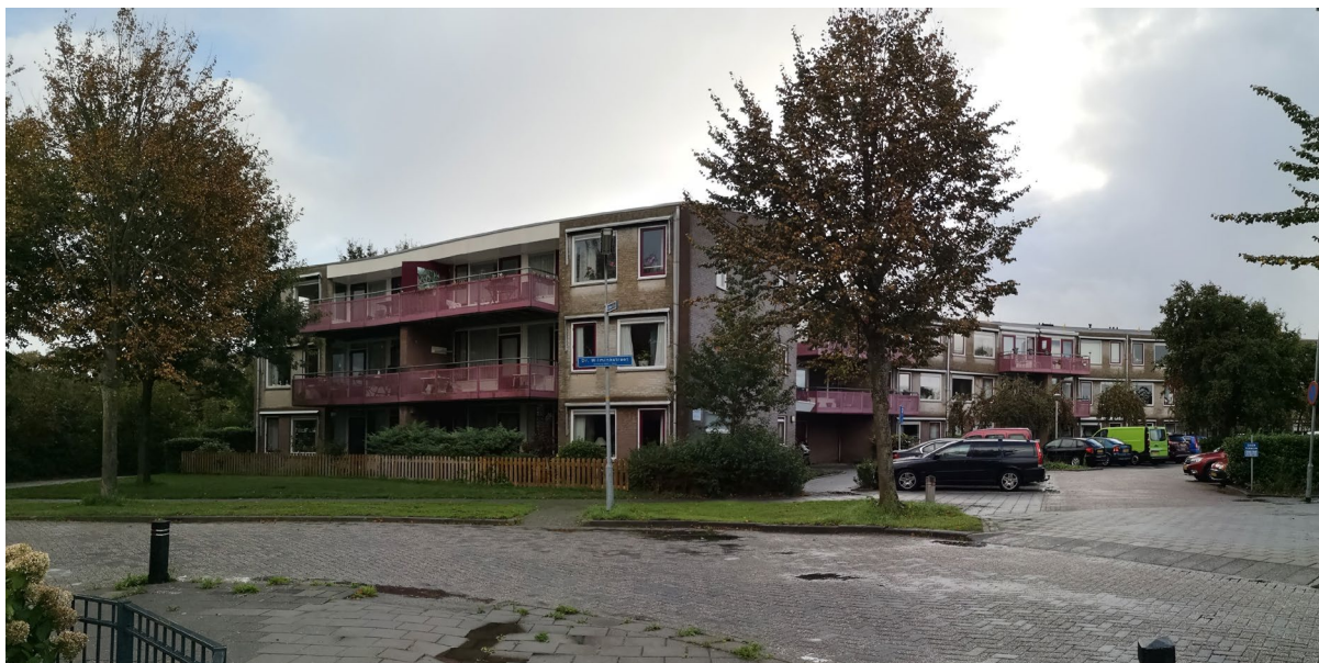
1 fig. 1.1.1: Exterior view at the complex at Zuid-Scharwoude (own image)
