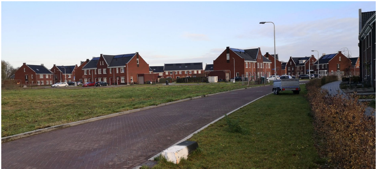
2 fig. 6.3.2: project location seen from east side, with access street towards surrounding neighborhood
