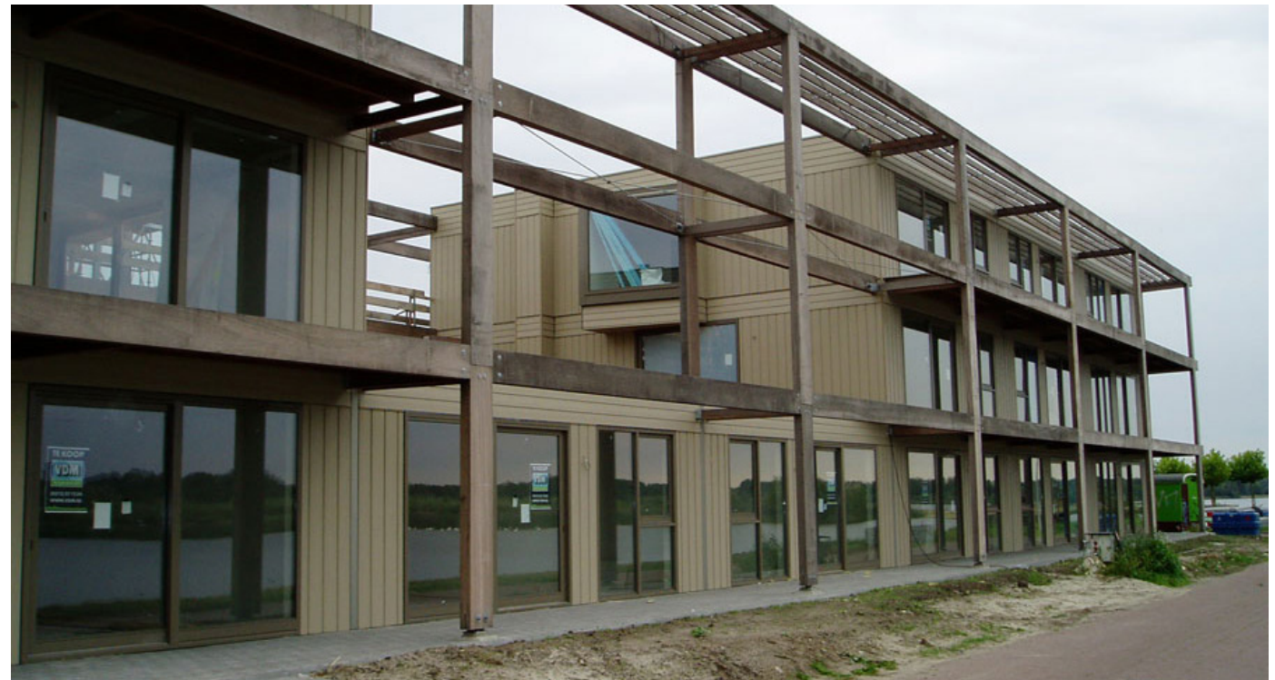
Wooden balconies and framing, Housing complex Borchrijk, Harkstede
