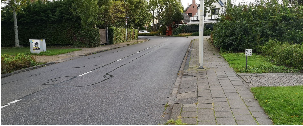
fig. 1.2.3: Dangerous, diagonal crossing of the road. (own image)
