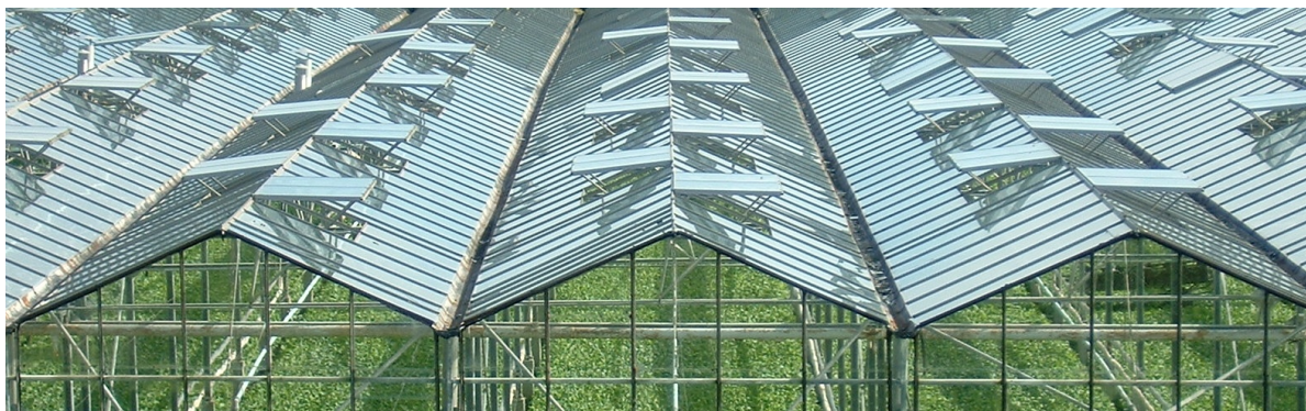
Figure 2.2: An example of a typical Venlo-style greenhouse. 2
