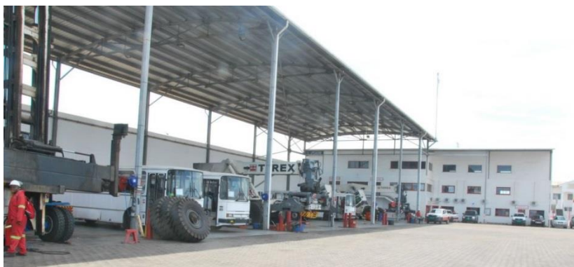
Figure 4-9: Impression maintenance hangar outside (Congo Terminal, 2016)
