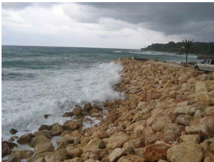
Figure 4-7: Impression revetment (Cummins and Cederberg, 2016)
