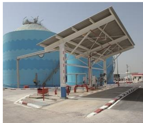
Figure 4-11: Impression terminal fuel facility (Kosan Crisplant, 2016)
