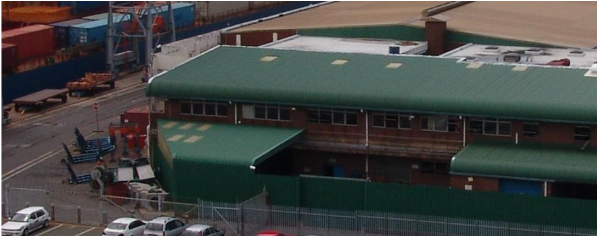
Figure 4-8: Impression operation building (South Africa, 2016)
