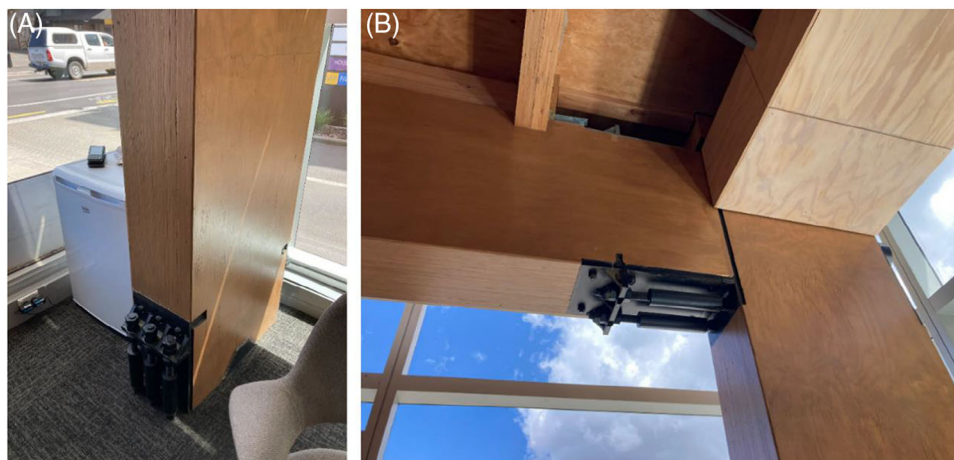
FIGURE 2 Example of (A) column-to-foundation connection and (B) beam-column connection with external damping devices, Young Hunter House, 'Merritt Building', Christchurch (NZ) (pictures courtesy of G. Formichetti).
