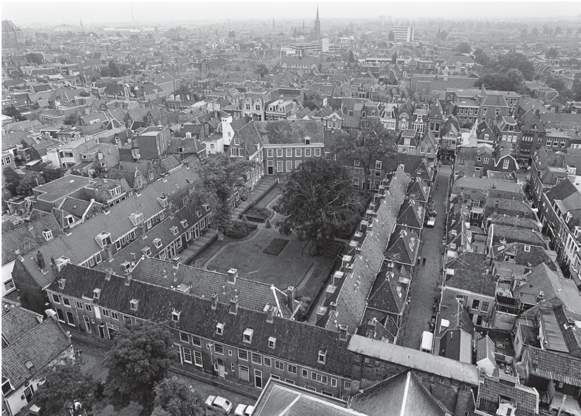
Figure 6: The Proveniershuis in Haarlem, photo taken in 1978, source: Delft Architectural Studies on Housing, Proveniershof Haarlem (NL), Dash2018/June, P82
