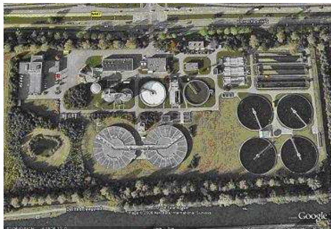
Figure 3-9 – Photograph of the Leiden Zuidwest WWTP
