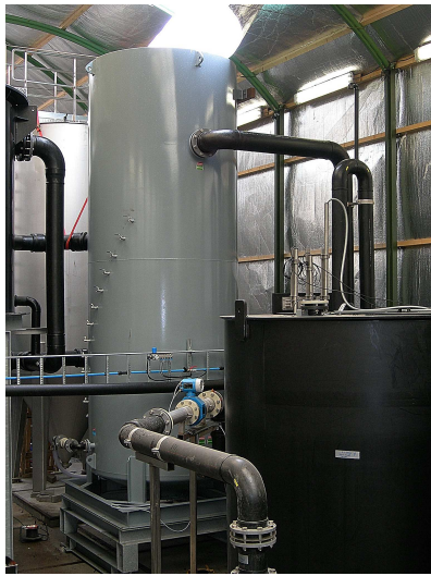
Figure 3-13 – Photograph of the dual media filter at the Leiden Zuidwest WWTP
