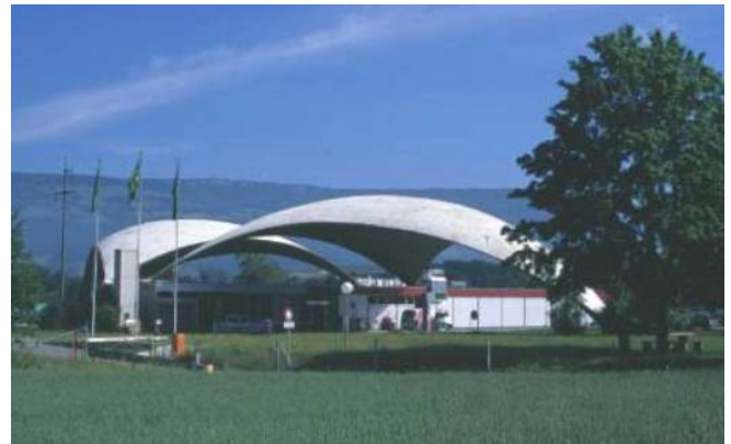
(a) - A thin concrete shell. Service station in Deitingen-Süd, Switzerland, designed by Heinz Isler.
