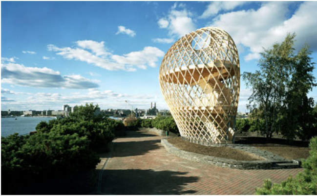
(a) - Korkeasaari Island Lookout Tower, Helsinki, Finland. Timber grid shell. Designed by Avanto Architects.
