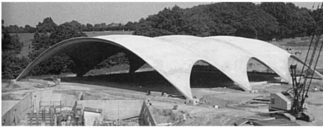
(a) - Indoor Tennis Center, Heimberg, Switzerland, 1978. A thin shell structure, designed by Heinz Isler.
