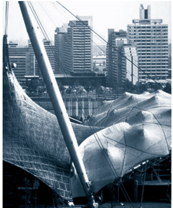
(b) - Roof of the Olympic Stadium, Munich, Germany, 1972. A membrane steel structure, designed by Frei Otto.
