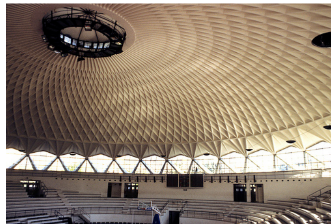
Figure 3.13 - Palazzetto dello Sport, a ribbed concrete shell, designed by Pier Luigi Nervi (Rome, Italy, 1957)
