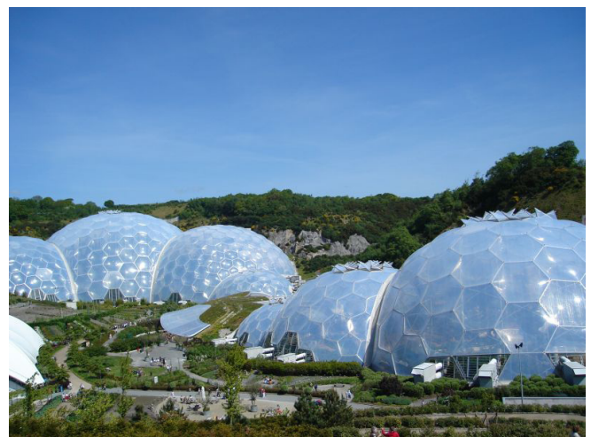
(b) - The Eden Project, Cornwall, UK. Steel grid shells by Nicholas Grimshaw.
