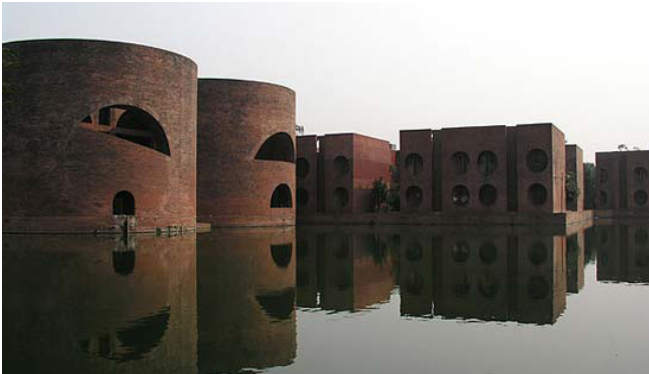
Brick buildings in Dhaka, Bangladesh. Design by Louis Kahn.
