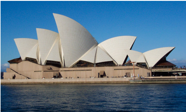
(b) - Sydney Opera House, Australia, 1973. Concrete frame & precast concrete ribbed roof. Engineered by Arup.
