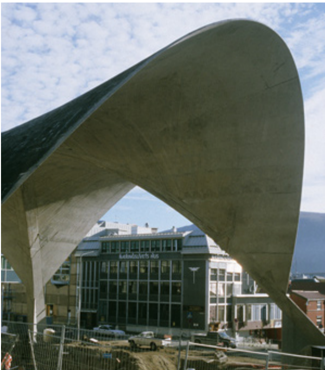
(c) - Roof of the 'Central Library' during construction, Tromsø, Norway, 1970. Designed by Gunnar Bøgeberg Haugen.
