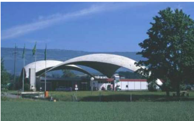
Figure 3.16 - A service station in Deitingen-Süd (Switzerland). A bubble shell, designed by Heinz Isler
