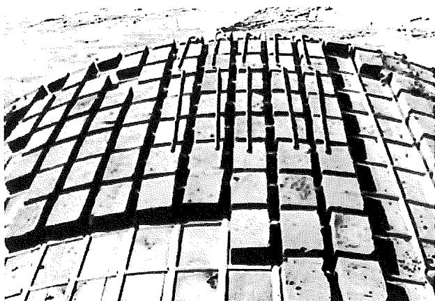
Figure 6.2 - Wooden formwork to construct the structures of Eladio Dieste
