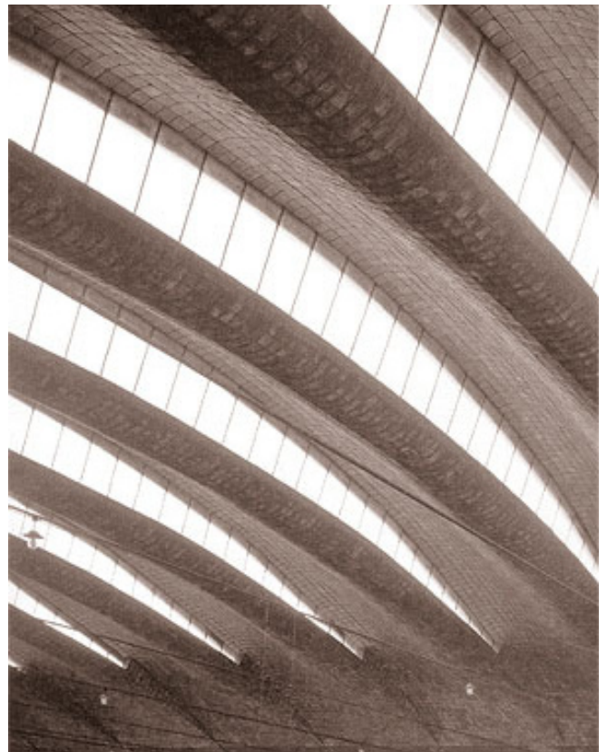
(f) - Roof of 'Julio Herrera & Obes Warehouses', Montevideo, Uruguay. Completed in 1979.
