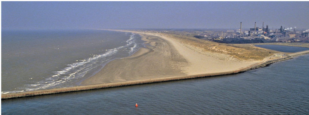
Figure 2.14: Picture taken in 1993 showing the coastline north of the port of IJmuiden, which clearly shows the large sedimentation area next to the breakwater. (source https://beelddbank.rws.nl/ )
