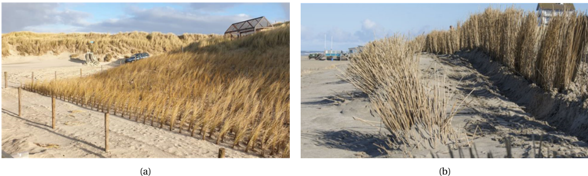
Figure 1.3: Maintenance works by HHNK to trap sediment in front of the dunes by planting grass (panel a, source: HHNK) and by placing reed fences (panel b, source: Staatsbosbeheer).
