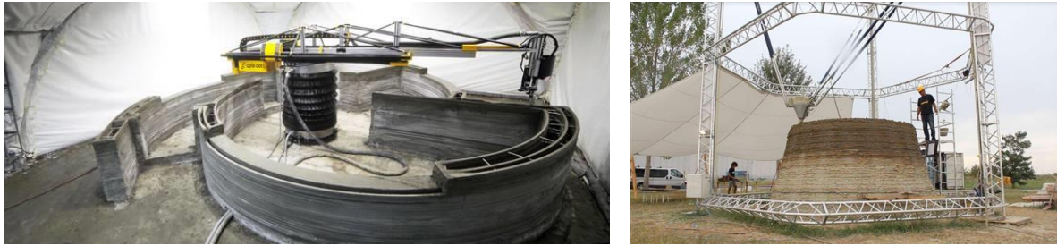
FIGURE 15 APIS COR HOUSE (OUTSIDE THE BOX) (CORBOY, 2017), WASP PROJECT ITALY (INSIDE THE BOX) (WANG, 2016)
