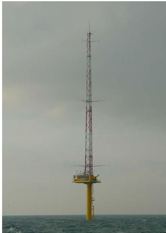
Figure 3.2: The mast and the installation of booms [39]
